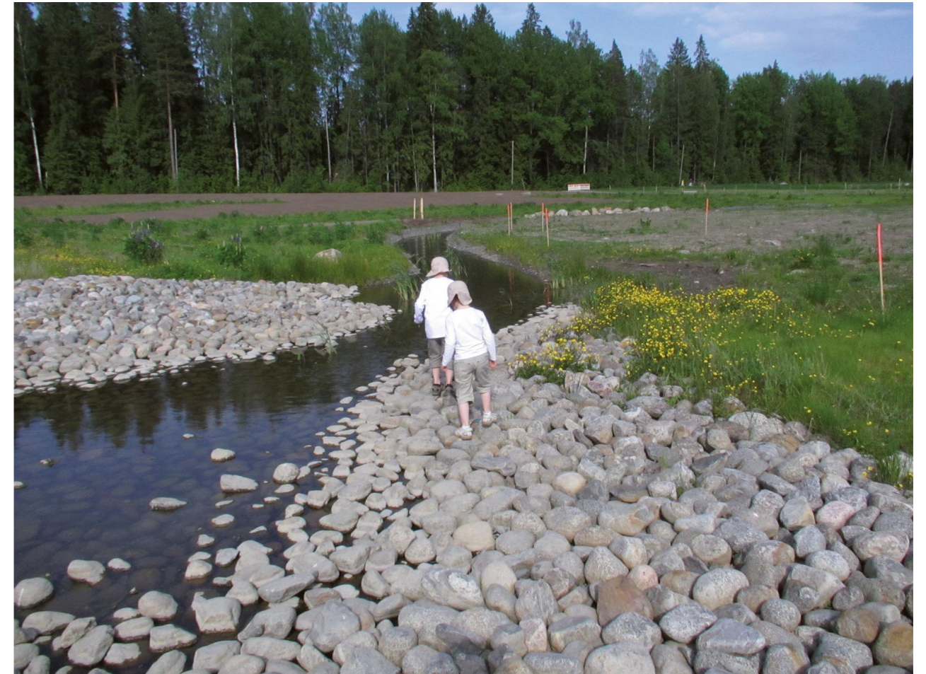
Image 53. Natural drainage systems are being actively developed in Tampere. For example, one of the largest drainage areas in Finland, which also serves as a recreational area for residents, has been built in Vuores. Water quality and flow are monitored by automatic measurements throughout the year. Measurements provide information on the ability of the current drainage system to purify drainage water and to reduce flows. The Urban Nature Labs project piloted urban drainage water management through nature-based systems in collaboration with city residents throughout the city, for example in Hiedanranta. Image: City of Tampere.
