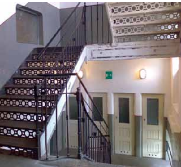
In industrial lofts, closets were often located in staircases, such as here in the old Finlayson Cotton Mill. © Seija Linnanmäki, 2010.
