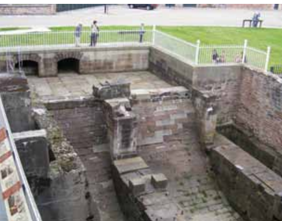
Stanley Mills, showing the wheelpits, with curved stonework that guided water onto two breastshot waterwheels, built in 1823–5, filled in since 1922 and excavated by Historic Scotland in 1995–8. There were two further wheels in tandem beyond these. The power take up went separately into Bell and Mid Mills. The concrete casing for a water turbine stands in the left hand wheel pit, put in after the eccentric working of the wheels had distorted the stone surrounds. © Mark Watson 2010.
