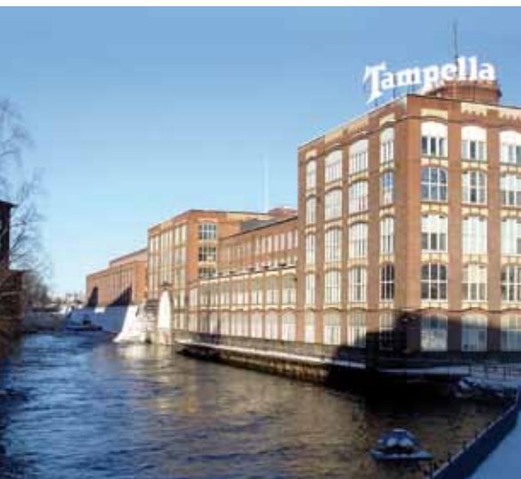
The old linen factory and engineering workshop buildings of Tampella. © Mikko Järvi.
