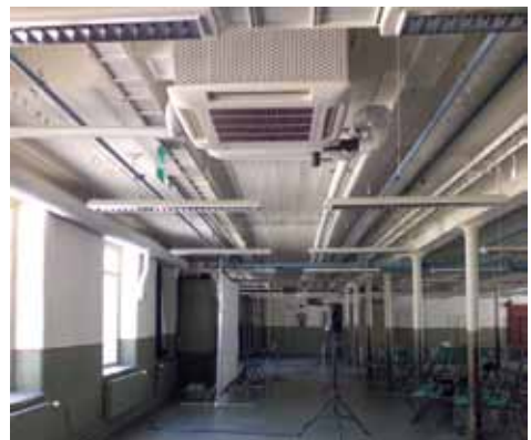
Old downward facing sprinkler heads were supplemented by new pipes and sprinkler heads facing upwards. Renovation Architect Studio Lasse Kosunen 2005. © Seija Linmanmäki, 2010.
