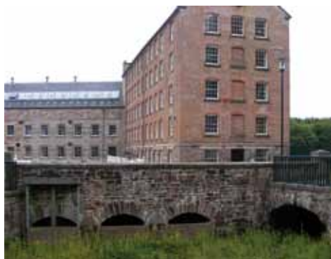
Stanley Mills, Scotland, showing the original Bell Mill, of 1786–7, Arkwright pattern on the right and Mid Mill, three phases from 1823–1840, on the left. Three stone arches carried water to the wheels, and the fourth led to an earlier corn mill and spillway. © Mark Watson 2010.
